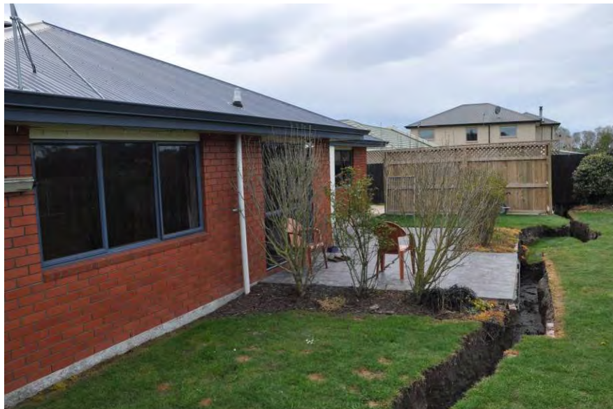
Figure 5.20 Ground failure feature extending through the backyard of a house on the south side of Courtenay Dr in the South Kaiapoi residential community. (-43.3894°, 172.6633°; 1500 hrs on 11 September 2010)
