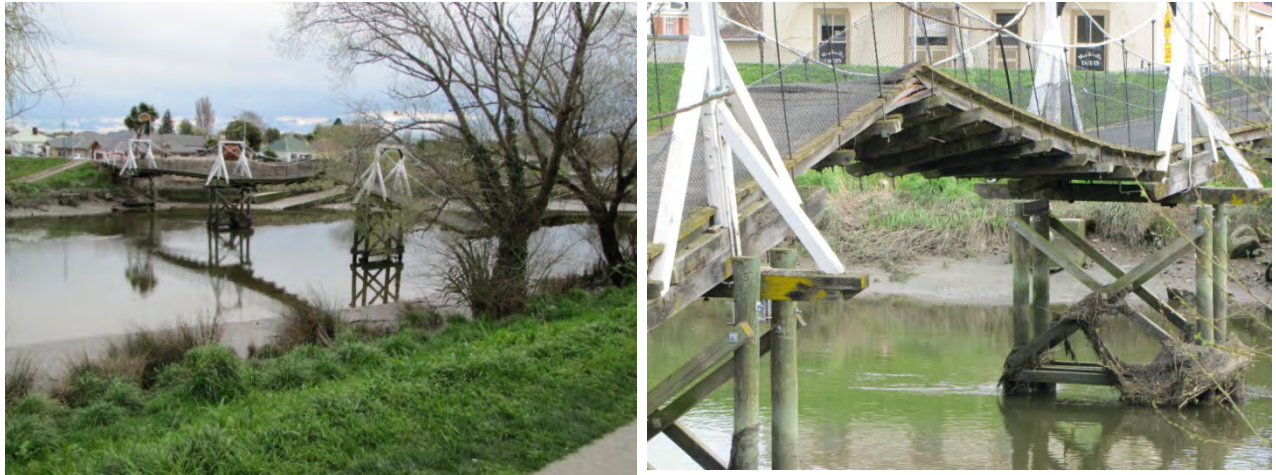
Figure 7.19 Buckling of footbridge near Trousselot Park. ( -43.3811^{\circ} , 172.6558^{\circ} )
