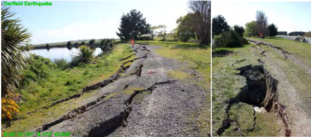
Figure 6.35 Lateral spread cracks at the eastern end of Pond 2B. The sinkhole in the foreground of the photo on the right formed over the top of two outlet pipelines. ( -43.52895^{\circ} , 172.717300^{\circ} )
