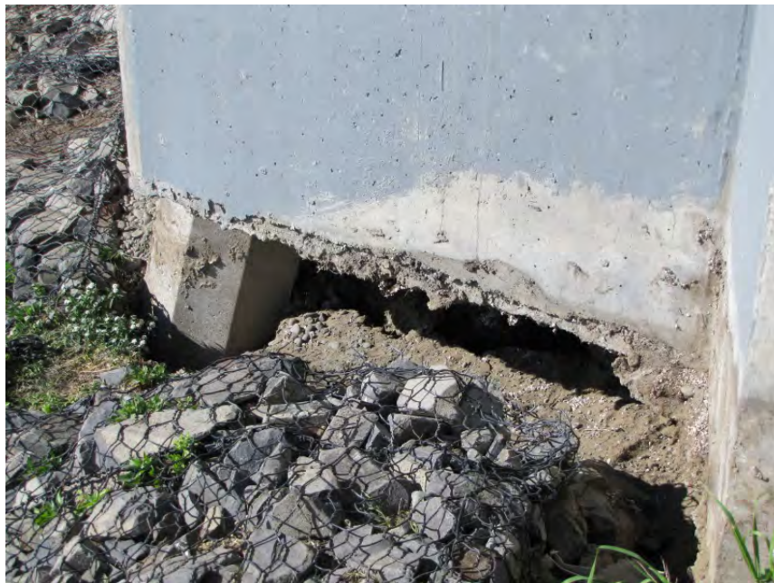
Figure 7.6 West abutment battered pile, Bridge Street Bridge. (-43.5253°, 172.7242°)
