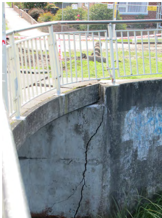
Figure 7.14 Cracking of north abutment, Swanns Road Bridge. ( -43.5222^{\circ} , 172.6600^{\circ} )
