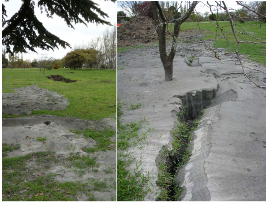
Figure 6.21 Photo 19 and 20: Lateral spread cracks along landside of the levee on the north side of the Kaiapoi River. The locations of these photographs are denoted in Figure 6.4. ( -43.384633^{\circ} , 172.661231^{\circ} )
