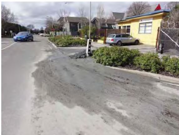
Figure 4.12 Evidence of limited/partial liquefaction in areas of Christchurch: (a) Evidence of liquefaction at Peterborough St - Madras St (CBD) ; (b) Sand boil in the foundation soils of a transmission tower (sub-station northeast of Greens Rd – Ruddenklau Ln, Bishopdale) (-43.4928055°, 172.5918055°).
