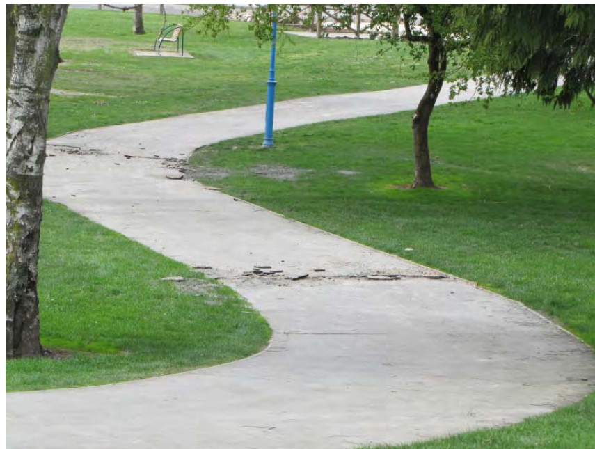
Figure 7.20 Cracking of sidewalk and evidence of liquefaction in Trousselot Park. ( -43.3811^{\circ} , 172.6558^{\circ} )
