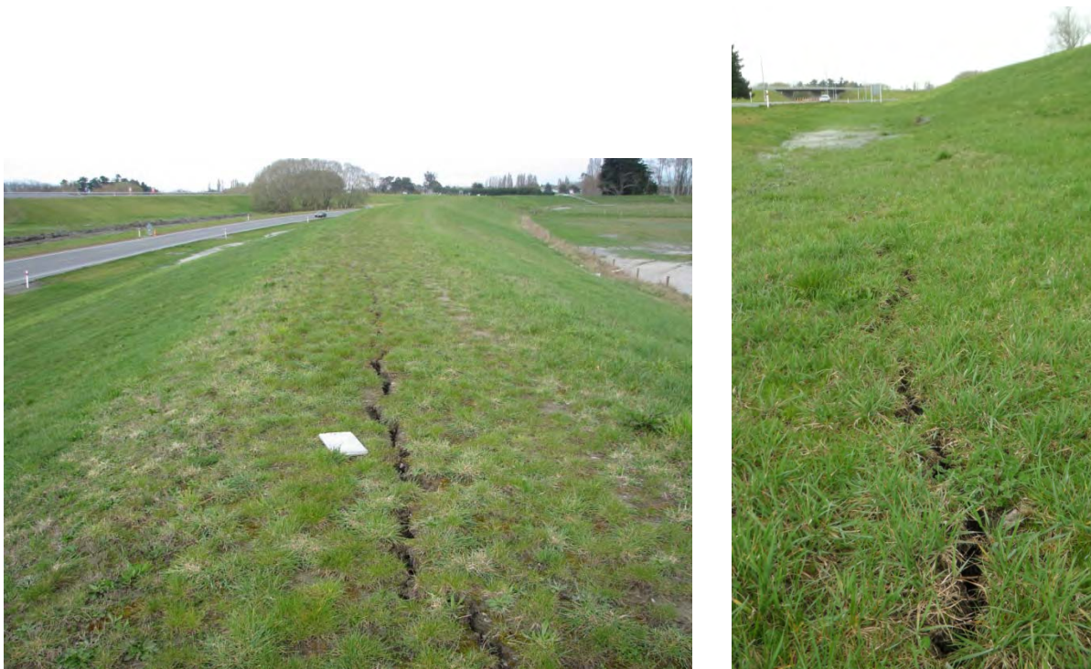
Figure 6.17 Photos 9 and 10: ~5-cm wide longitudinal cracks running along the crest (left) and base (right) of a secondary levee for the Waimakariri River. Photo taken looking southwest; SH1 on left of levee. The locations of these photographs are denoted in Figure 6.4. (-43.430108°, 172.643434°)
