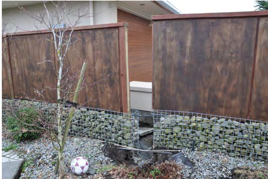
Figure 5.48 Separated fence line due to propagating ground fissure meandering between houses along Riverside Ln. (-43.43096°, 172.6931°; 1230hrs on 13 September 2010)
