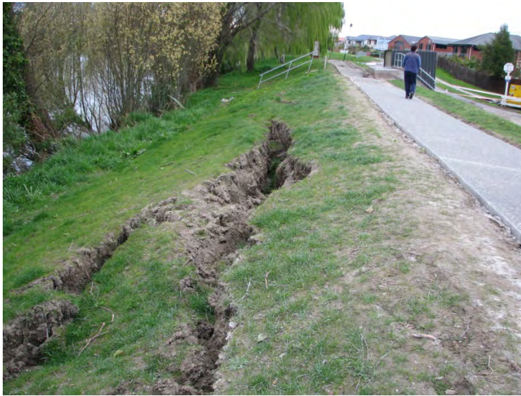
Figure 6.25 Photo 25: Lateral spread cracks along riverside levee on the south side of the Kaiapoi River. The location of this photograph is denoted in Figure 6.4. (-43.385254°, 172.660131°)
