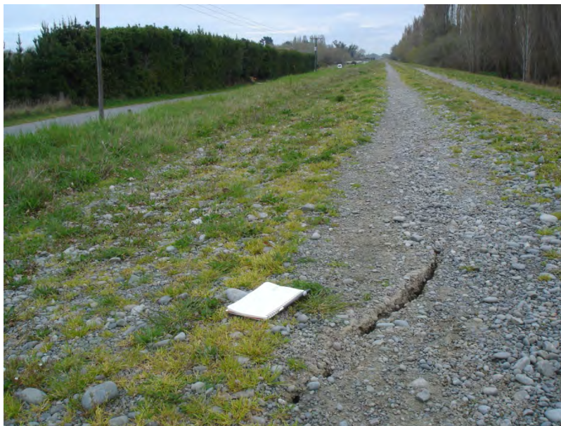
Figure 6.10 Photo 5: ~2-cm wide crack running lengthwise along the top of the levee on Coutts Island Rd. This crack was at the edge of the ~0.5 km stretch of the levee where significant liquefaction was observed. Photo taken looking southwest. The location of this photograph is denoted in Figure 6.4. ( -43.423440^{\circ} , 172.632349^{\circ} )
