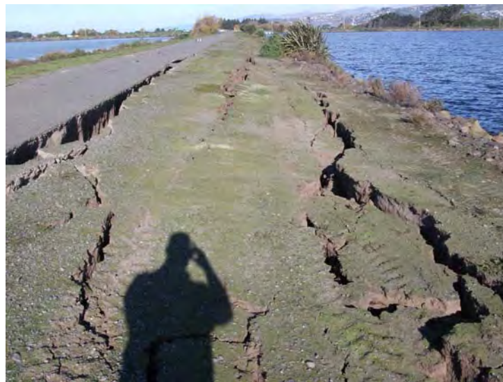
Figure 6.33 Lateral spread cracks running parallel to Dyers Road adjacent to Pond 2A. ( -43.531393^{\circ} , 172.712473^{\circ} )
