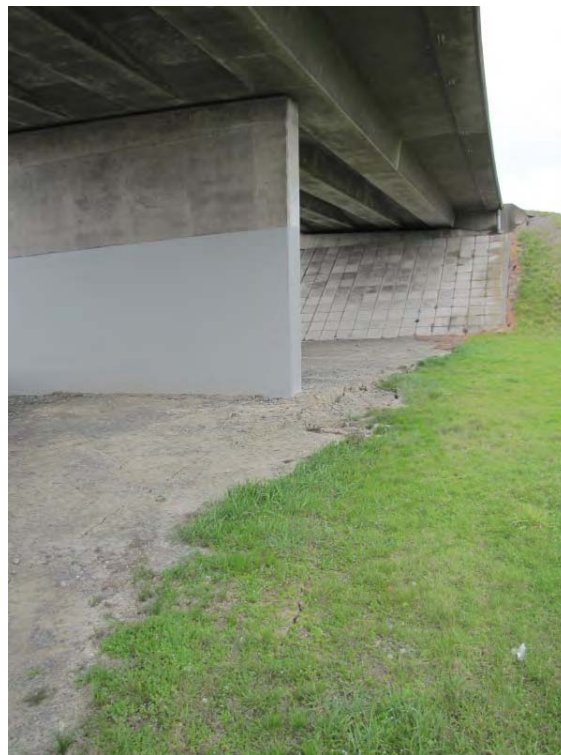
Figure 7.24 Evidence of liquefaction beneath Chaney's Overpass. (-43.4300°, 172.6464°)
