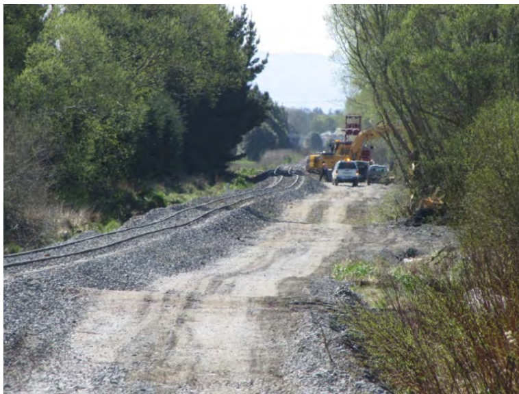
Figure 4.33 Damage to train tracks due to ground movement. (Position 3; -43.4068°, 172.6489°)
