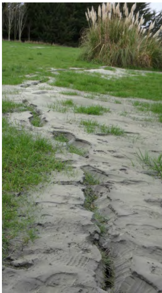
Figure 6.30 Liquefaction and lateral spread features on or near levees located about 100 to 200 m west of the Kaiapoi Sewage Treatment Plant. (upper left: -43.389175^{\circ} , 172.683235^{\circ} ; upper right: -43.389701^{\circ} , 172.683390^{\circ} ; bottom left: -43.389519^{\circ} , 172.682203^{\circ} ; bottom right: -43.389432^{\circ} , 172.6682060^{\circ} )
