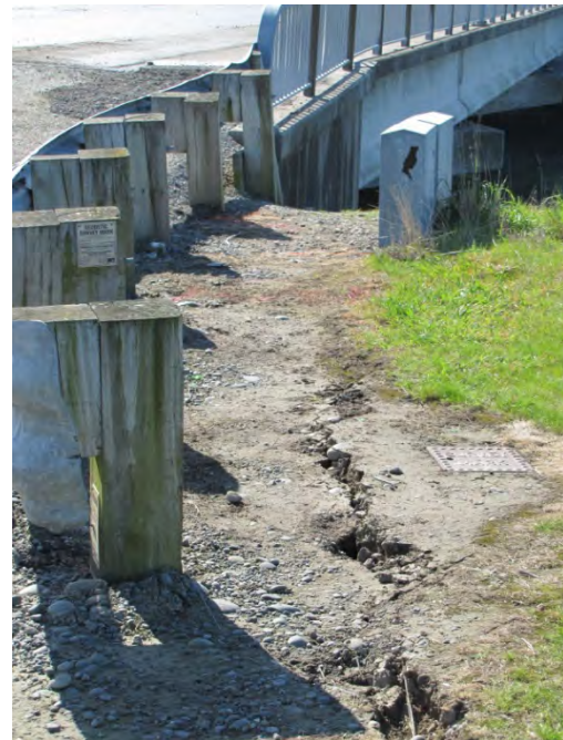
Figure 7.2 Cracking on margins of west approach embankment, Bridge Street Bridge. (-43.5253°, 172.7242°)
