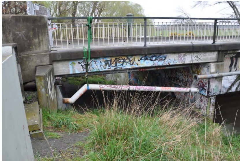
Figure 7.31 Damage to sewage pipe at the Kainga Road Bridge ( -43.3997^{\circ} , 172.6916^{\circ} )
