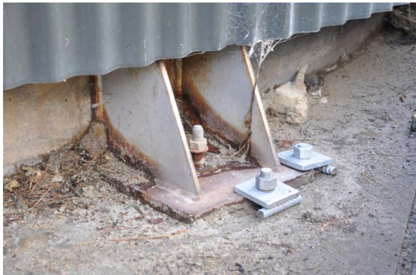
Figure 7.43 Typical repair to Tank 3 and 4 (addition of clamp plates). Note the pullout of the original anchorage. Fulton Hogan Bitumen Plant. (-43.6085°, 172.7149°).
