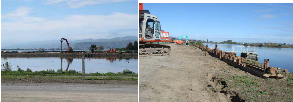
Figure 6.36 Sheet piles being driven to stabilize the pond embankment to arrest further movement. ( -43.530563^{\circ} , 172.718349^{\circ} )
