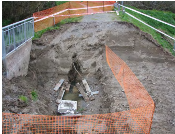
Figure 6.28 Photo 28: Failed drainage conduits running underneath the levee on the southside of the Kaiapoi River. The location of this photograph is denoted in Figure 6.4. (-43.388679°, 172.666203°)
