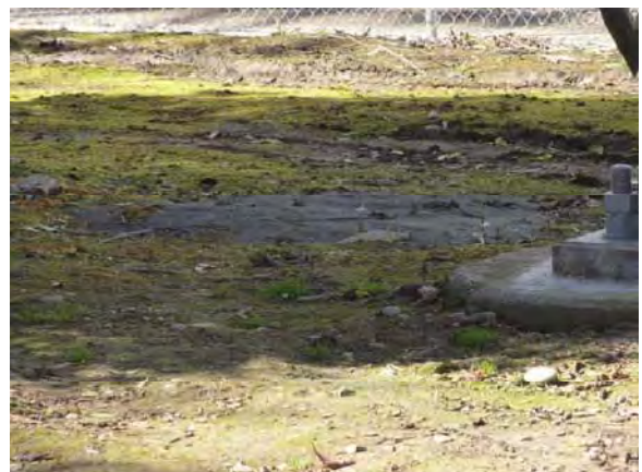
Figure 4.12 Evidence of limited/partial liquefaction in areas of Christchurch: (a) Evidence of liquefaction at Peterborough St - Madras St (CBD) ; (b) Sand boil in the foundation soils of a transmission tower (sub-station northeast of Greens Rd – Ruddenklau Ln, Bishopdale) (-43.4928055°, 172.5918055°).
