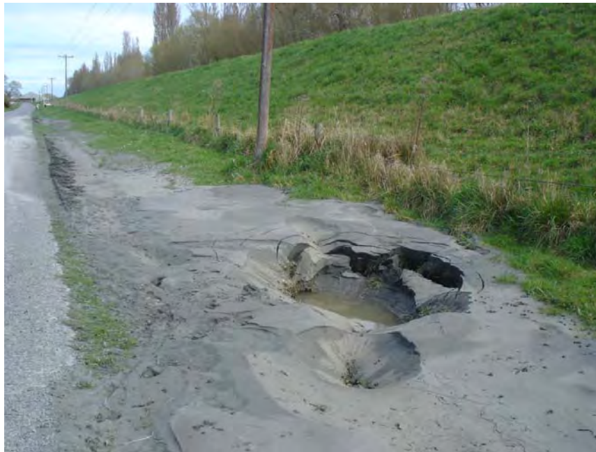
Figure 6.6 Photo 1: Large sand boil at the base of the landside of the levee on Coutts Island Rd. The location of this photograph is denoted in Figure 6.4. (-43.425018°, 172.628442°)
