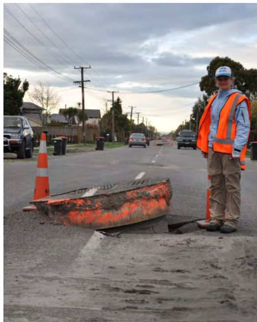
Figure 7.47 Uplifted manholes along Lower Styx Road, note the uplifted manholes in the background too. ( -43.4113^{\circ} , 172.6930^{\circ} ).
