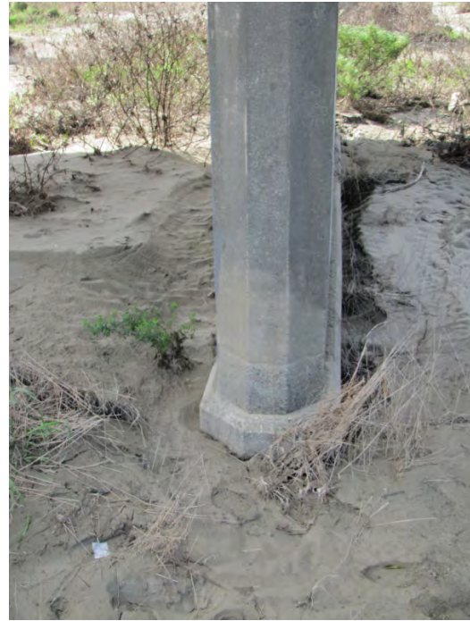
Figure 7.29 Evidence of liquefaction at Highway 1 bridge piers on the north side of the Waimakariri River. ( -43.4153^{\circ} , 172.6467^{\circ} )
