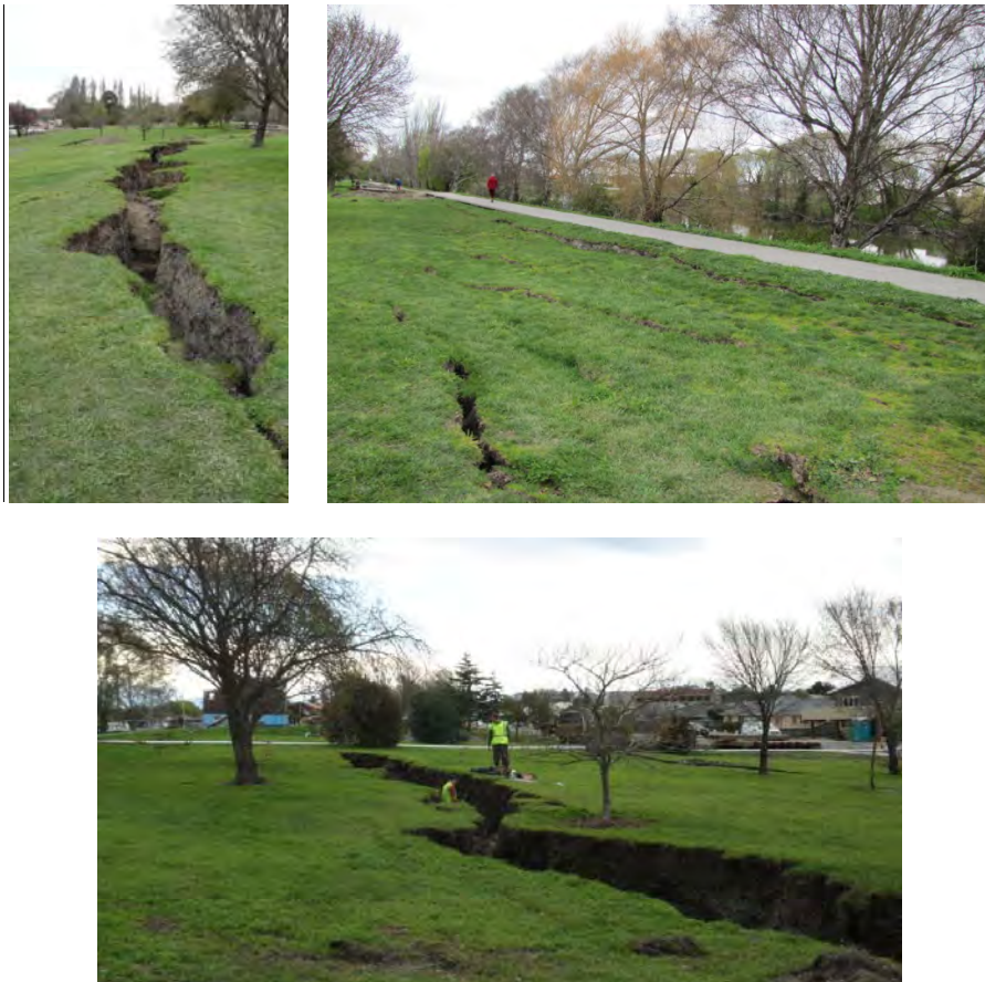
Figure 6.20 Photos 16-18: Lateral spread cracks along landside of the levee on the north side of the Kaiapoi River. The locations of these photographs are denoted in Figure 6.4. ( -43.384484^{\circ} , 172.660653^{\circ} )
