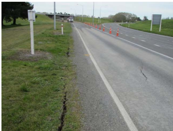
Figure 7.26 Cracking in and along roadway adjacent to Chaney's Overpass. ( -43.4300^{\circ} , 172.6464^{\circ} )
