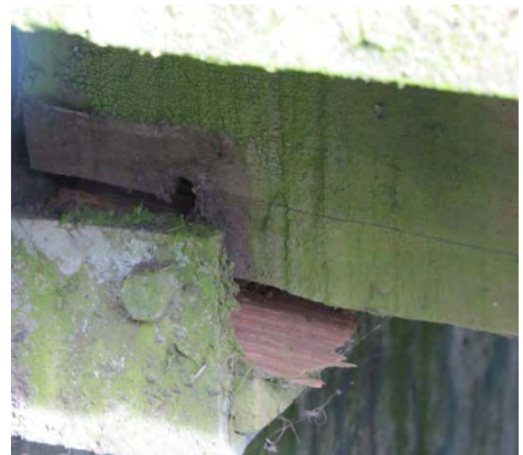
Figure 7.16 Footbridge on the Avon River near Medway Road: (a) Buckled span; and (b) Sheared bearing on east bank. ( -43.5310^\circ , 172.6656^\circ )
