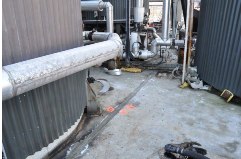
Figure 7.44 Repair of lateral spread cracks within the Fulton Hogan Bitumen Plant, nearby Tank 3. (-43.6085°, 172.7150°)
