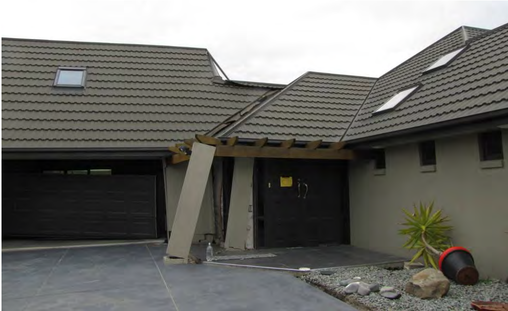
Figure 5.47. House with fissured floor slab with damage carried through to the roof line, which is no longer weather proof. (Riverside Ln, Spencerville). ( -43.4311^{\circ} , 172.6935^{\circ} ; 1600hrs on 28 September 2010)
