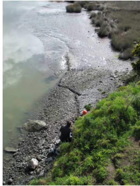
Figure 7.3 Lateral spreading of east banks adjacent to the Bridge Street Bridge. ( -43.5253^{\circ} , 172.7242^{\circ} )
