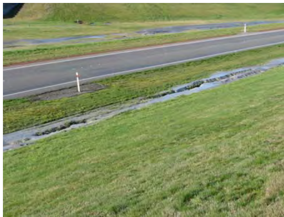
Figure 6.18 Photos 11 - 14: Liquefaction ejecta on both the river and landsides of the levee. The locations of these photographs are denoted in Figure 6.4. ( -43.428968^{\circ} , 172.645435^{\circ} )
