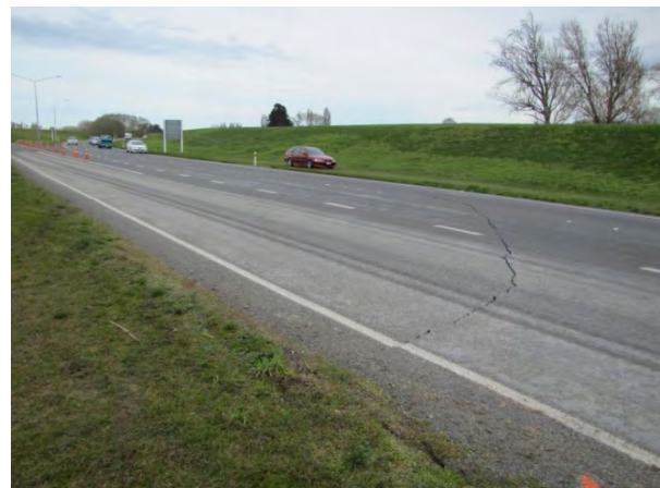
Figure 7.26 Cracking in and along roadway adjacent to Chaney's Overpass. ( -43.4300^{\circ} , 172.6464^{\circ} )
