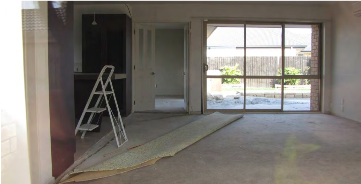
Figure 5.39. Fissure in concrete floor slab (to the left hand side passing beneath the ladder). (Same house as in Figure 5.38.) (Kokopu St; -43.5183°, 172.7220°; 1030hrs on 12 September 2010)
