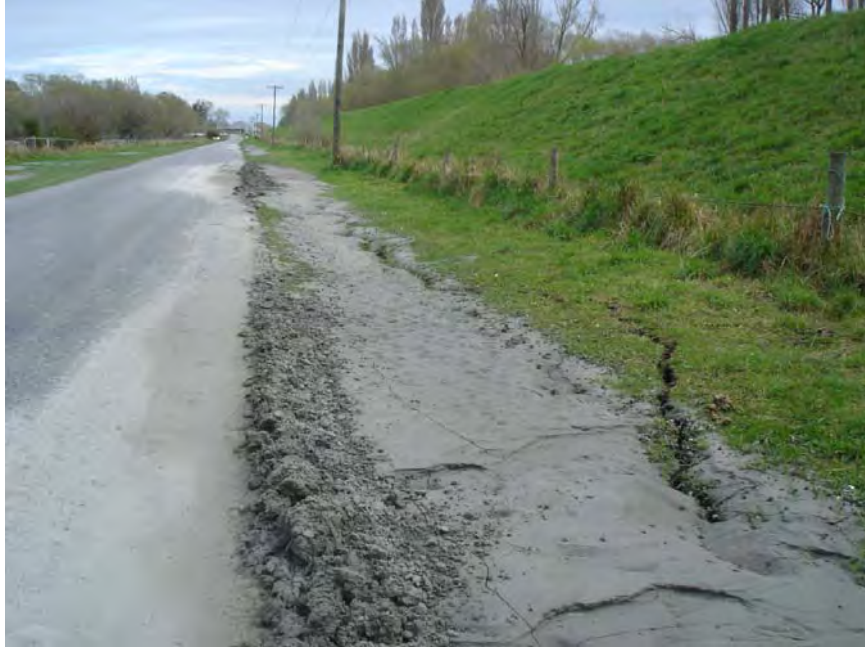
Figure 6.7 Photo 2: Crack running along base of levee on Coutts Island Rd (landside) and liquefaction ejecta. The location of this photograph is denoted in Figure 6.4. ( -43.424466^{\circ} , 172.629907^{\circ} )
