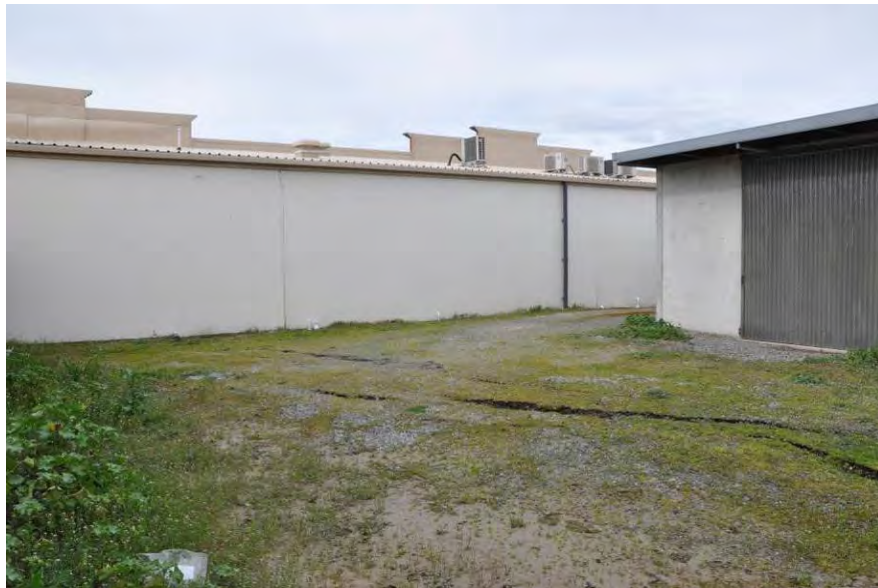
Figure 5.9 Surrounding ground failure patterns directly adjacent to the Property and Family Law Offices in Kaiapoi business district. View looking southeast ( 43.3819^{\circ} S, 172.6593^{\circ} E; 1100 hrs on 11 September 2010)
