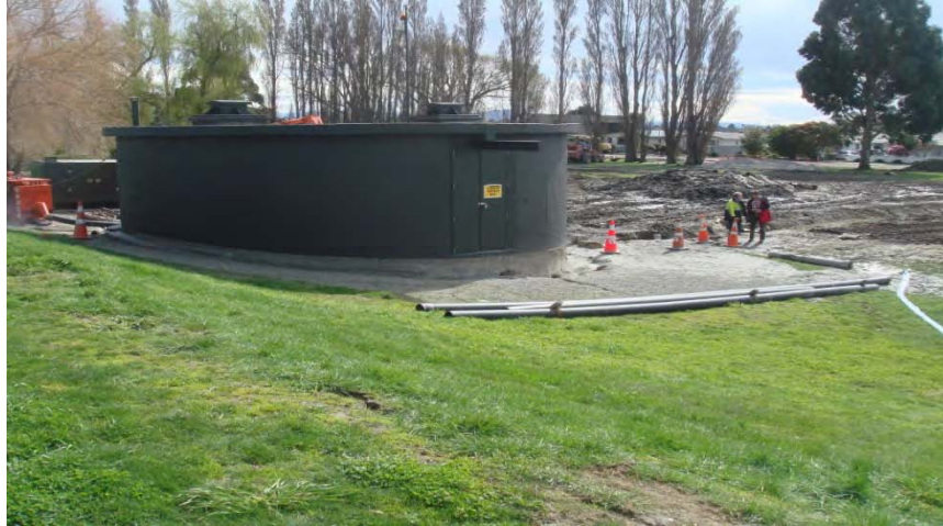
Figure 6.23 Photo 22: Tank that settled ~30 cm resulting in damage to attached pipes. The photograph numbers correspond to the locations denoted in Figure 6.4. ( -43.386918^\circ , 172.664412^\circ )
