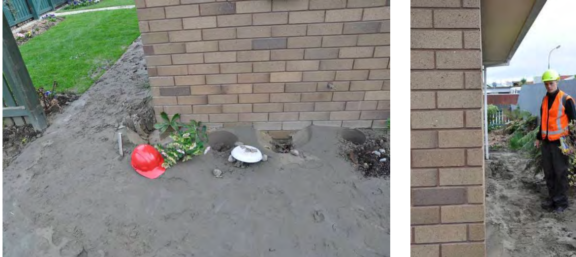
Figure 5.18 Red tagged residence on Charles St. Extensive surrounding ejecta at perimeter of house (43.3838°S, 172.6607°E; 1130 hrs on 11 September 2010)
