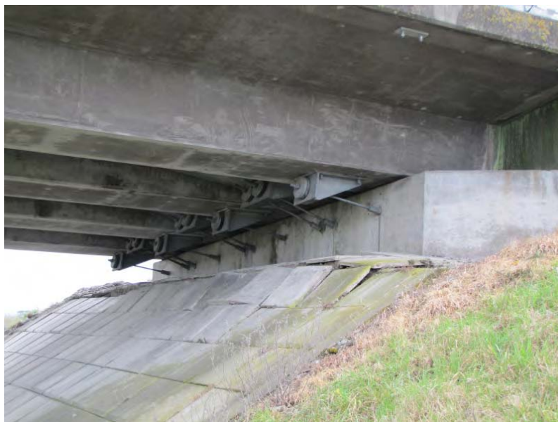
Figure 7.22 Cable Restrainers at north abutment, Chaney's Overpass. (-43.4300°, 172.6464°)
