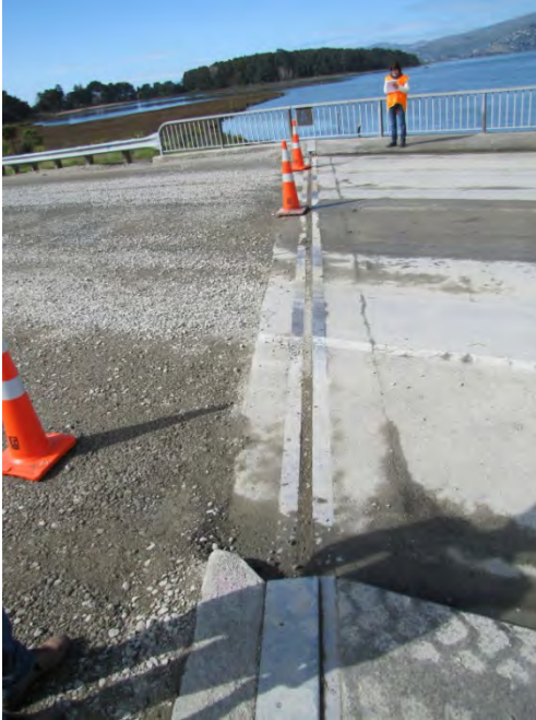
Figure 7.1 Repaired east approach to the Bridge Street Bridge. (-43.5253°, 172.7242°)
