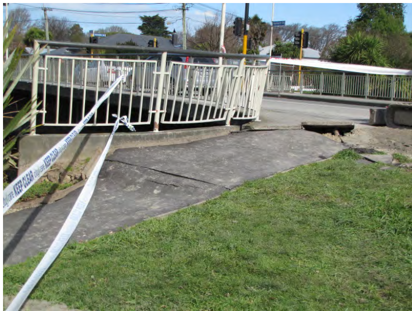
Figure 7.12 Incipient lateral spreading at west abutment, Swanns Road Bridge. ( -43.5222^{\circ} , 172.6600^{\circ} )
