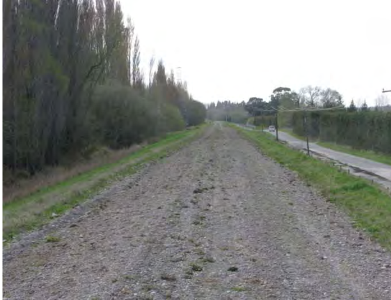
Figure 6.9 Photo 4: Road on top of levee that had recently been reggraded, presumably after the earthquake to fill in longitudinal cracks formed during the earthquake. Liquefaction was observed along the base of both sides of the levee along this stretch. The location of this photograph is denoted in Figure 6.4. ( -43.423943^{\circ} , 172.631045^{\circ} )
