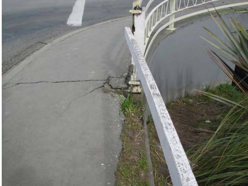
Figure 7.13 Incipient lateral spreading at north abutment, Gayhurst Road Bridge. ( -43.52172^{\circ} , 172.6728^{\circ} )
