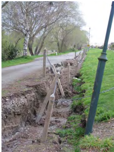
Figure 6.26 Photo 26: Lateral spread cracks along riverside levee on the south side of the Kaiapoi River. The location of this photograph is denoted in Figure 6.4. (-43.385839°, 172.660941°)
