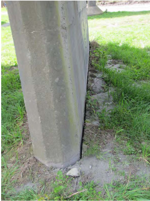
Figure 7.29 Evidence of liquefaction at Highway 1 bridge piers on the north side of the Waimakariri River. ( -43.4153^{\circ} , 172.6467^{\circ} )
