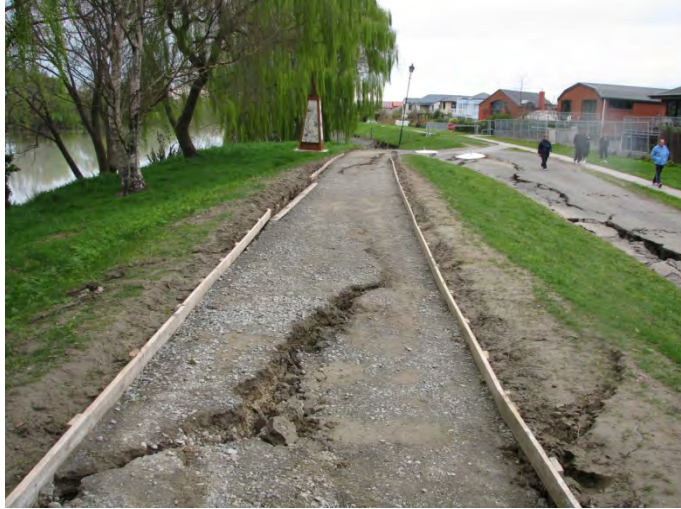
Figure 6.27 Photo 27: Lateral spread cracks along the top of the levee on the south side of the Kaiapoi River. The location of this photograph is denoted in Figure 6.4. (-43.385693°, 172.660688°)
