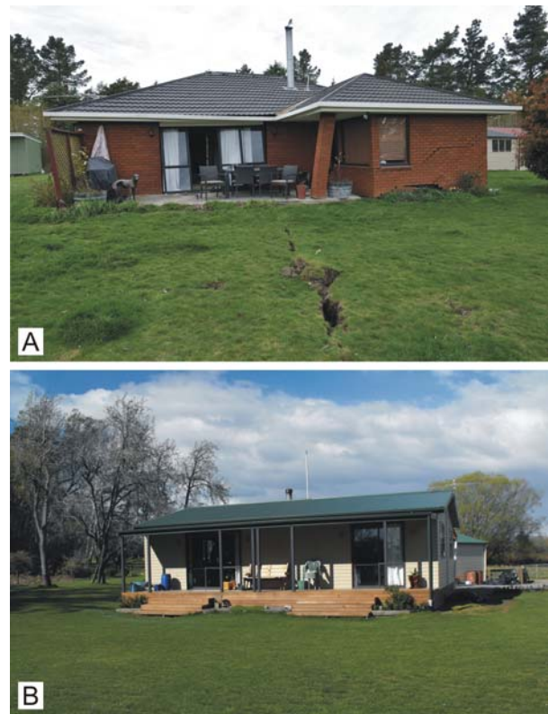
Figure 4. Examples of houses affected by Greendale Fault surface rupture. A) Timber-framed, brick-clad house with concrete slab foundation and light-weight roof that is located within a ~150 m wide deformation zone accommodating 4 to 5 m of dextral displacement. House is badly damaged by ~0.5 m of discrete strike-slip rupture that passes through the foundation of the house as well as distributed shear within the broad deformation zone. Photo by Dougal Townsend. B) Light-gauge steel framed, plywood- and weatherboard-clad house with steel pile foundation and steel I-beam bearers that is tilted, and rotated, but only slightly damaged, by ~1 m of distributed vertical and dextral fault rupture spread over several tens of metres width. Photo by Russ Van Dissen.
